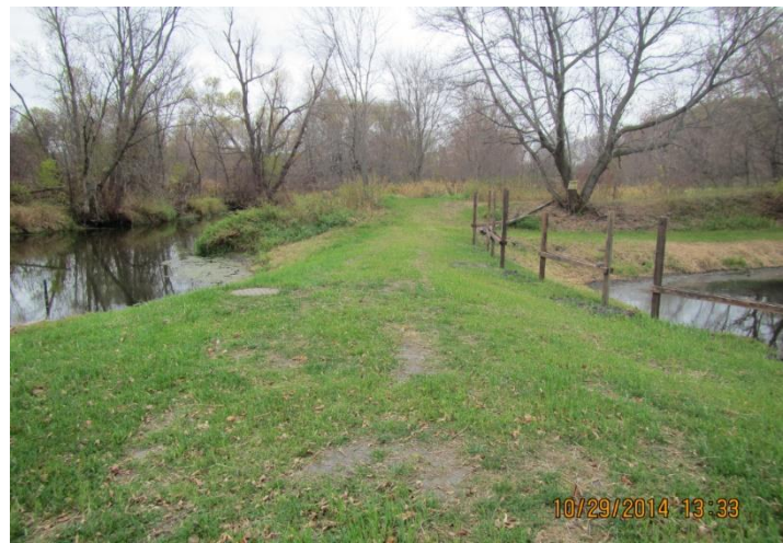
FIGURE 2 BERM AND INJECTION POINT AT DESILT POND
