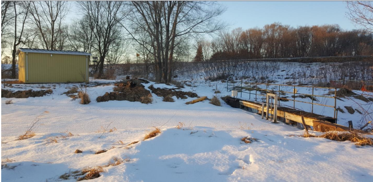
FIGURE 1 FERRIC CHLORIDE SHED AND WEIR
