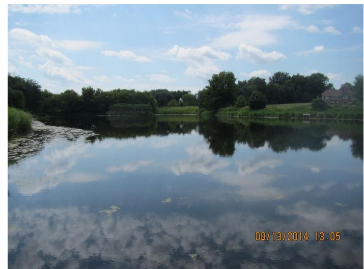
FIGURE 4 DESILT POND, STANDING AT OUTLET
