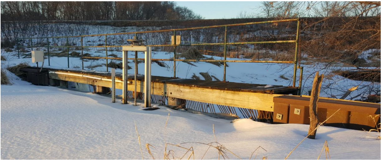
FIGURE 9 FERRIC CHLORIDE WEIR AND FISH BARRIER
