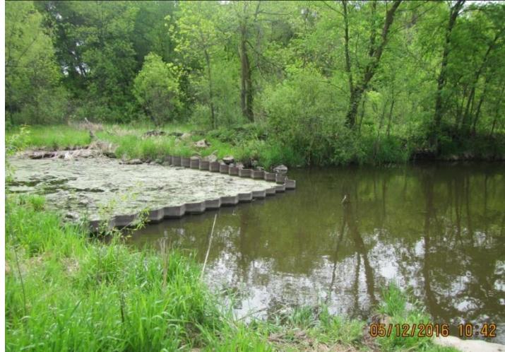
FIGURE 3 BYPASS WEIR AT DESILT POND
