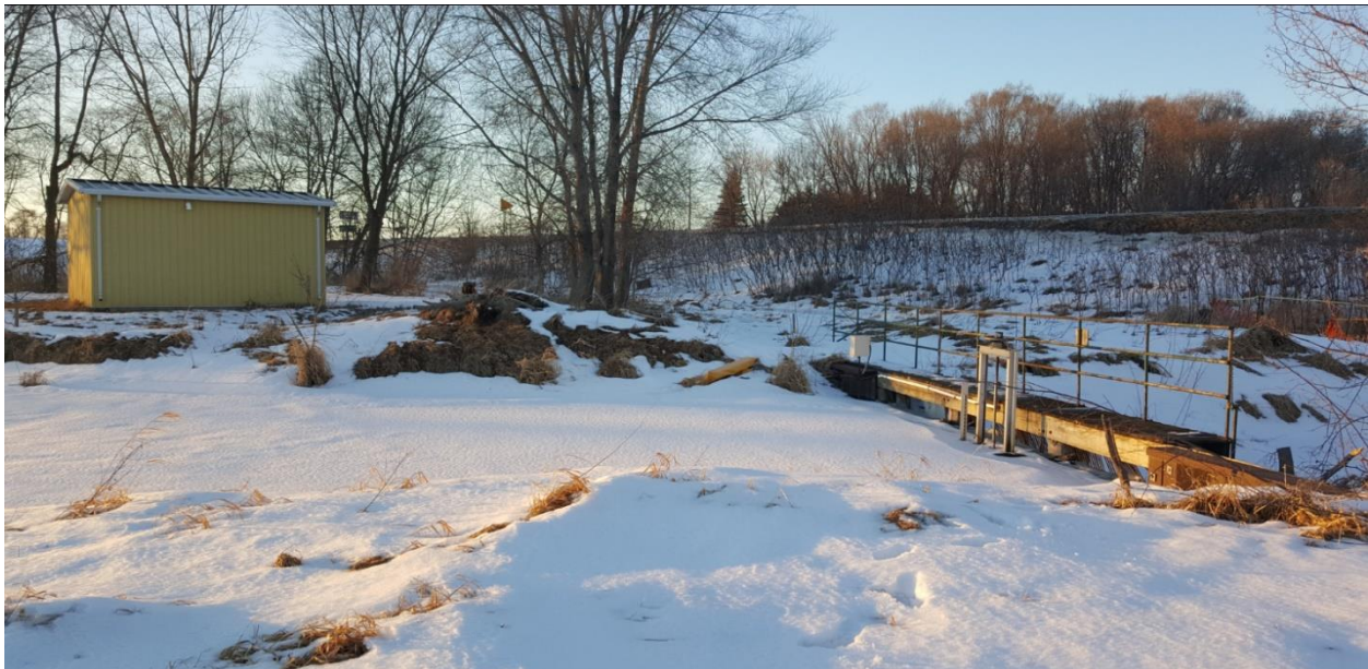
Figure 1. Ferric Chloride Shed and Weir
