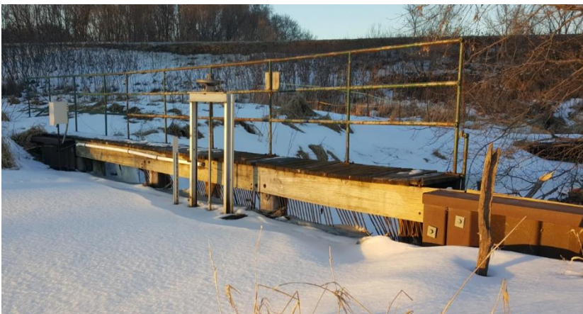
Figure 6. Ferric Chloride Weir and Fish Barrier
