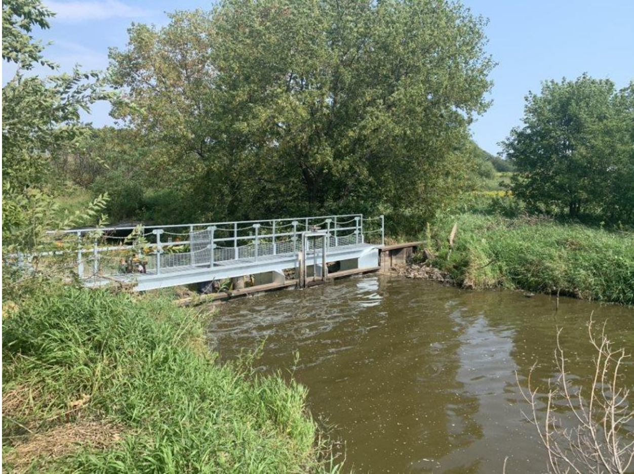
Figure 4 New walking deck over weir and fish barrier
